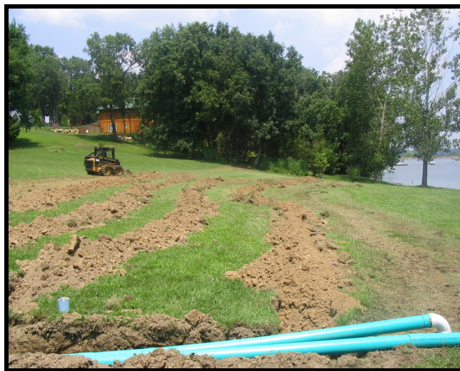
Dispersal trenches installed on contour.
