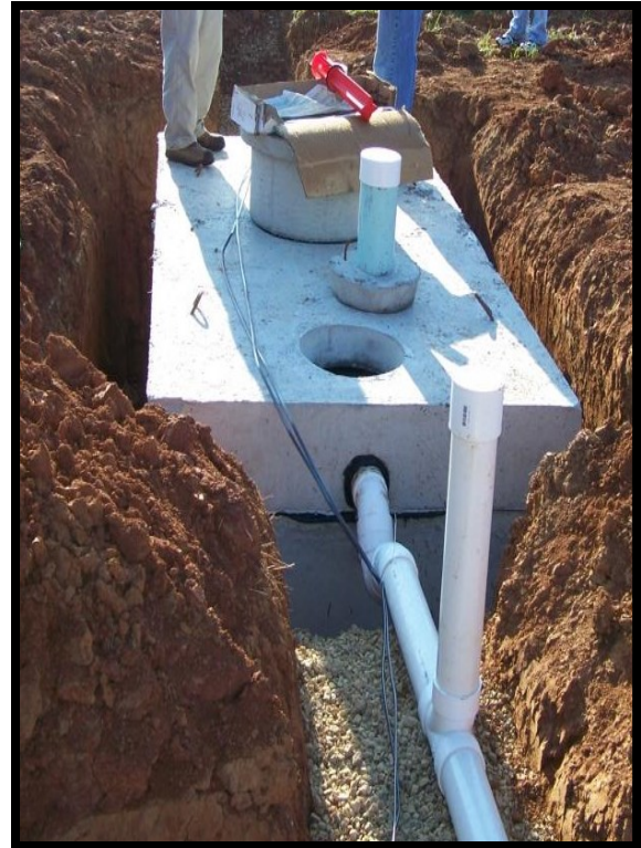
Installation of a 1,000 gallon concrete septic tank.
