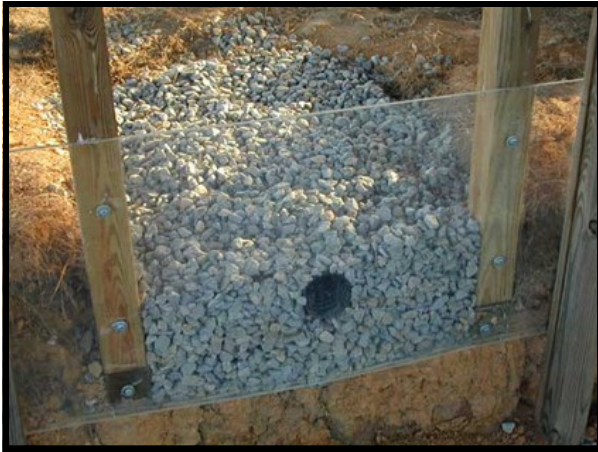
Conventional gravel trench with 4" inch perforated pipe.
