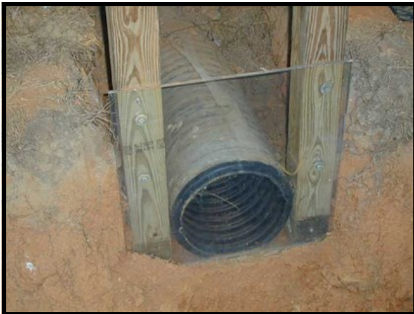
Filter wrapped 10" inch perforated corrugated pipe.
