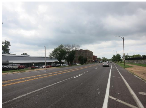
Broadway Looking South (Photo Taken on August 2, 2024)
