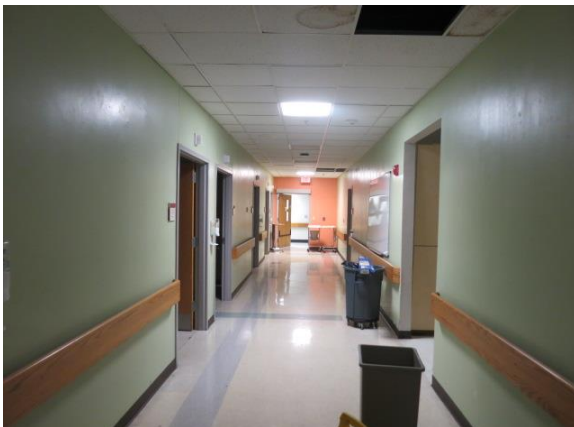
Interior View (Photo Taken on August 2, 2024)
