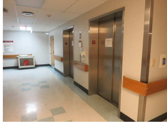
Interior View (Photo Taken on August 2, 2024)
