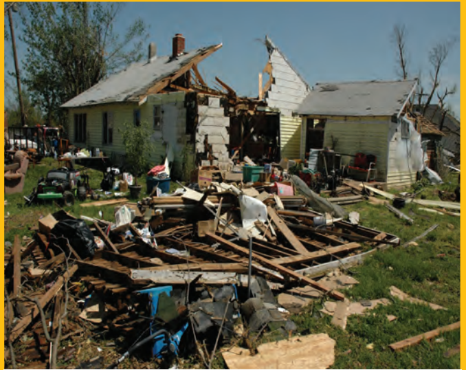
PHOTO: Newtonia, Missouri, May 12, 2008 -- An EF4 tornado cut a swath across southwest Missouri on May 10, badly damaging and destroying dozens of homes in Newtonia. Michael Raphael/FEMA
