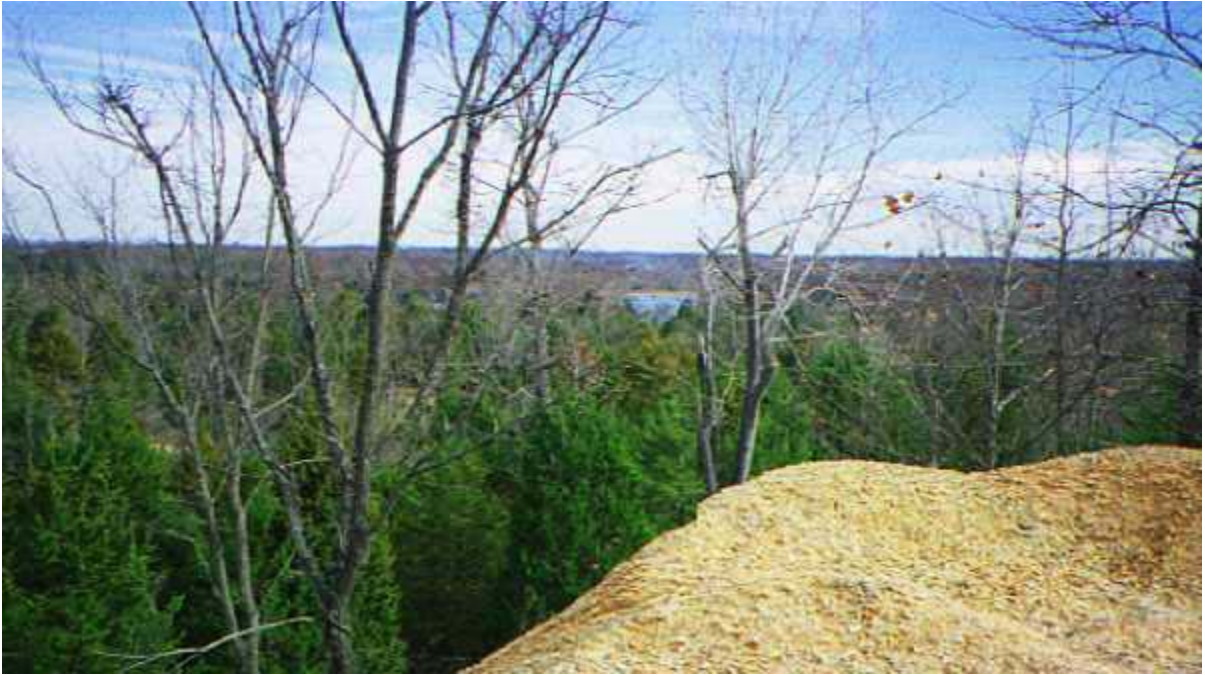
View of lake through tree cover, facing northeast toward landfill from the bottom of the tailings pond dam
