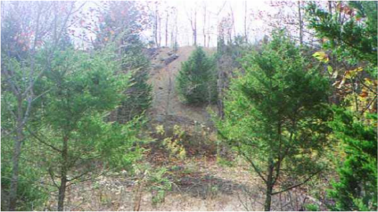
Side of tailings pond dam for De Soto Mining Company, Inc.
