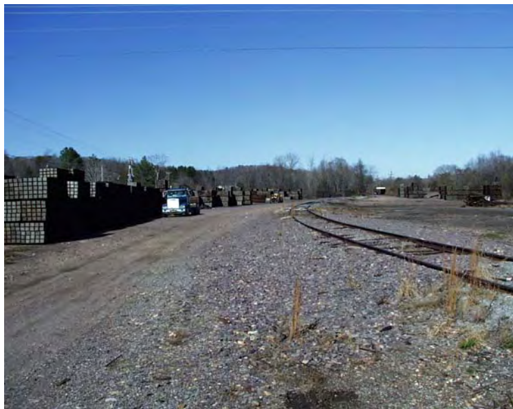
Figure 2. Picture of Vulcan Tie Yard to the north.
